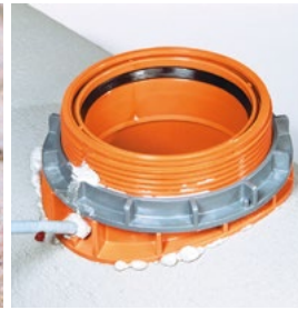
With a cartridge and a mixing tube, the resin can be filled in directly via the filling opening in the distance ring.
