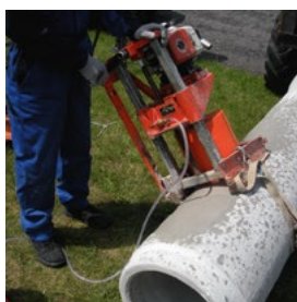
Correct Coredrilling
