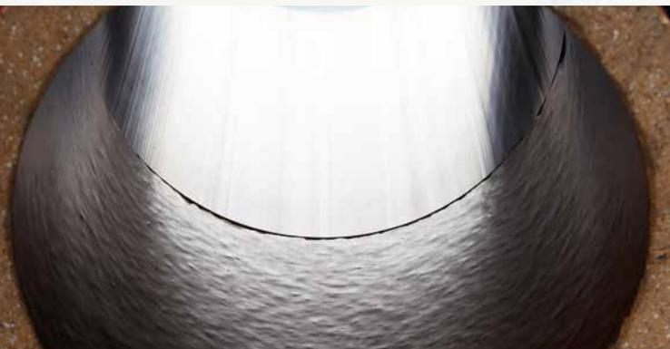
*The internal diameters of the PVC-U pipes match those of the clay or concrete pipes.*
