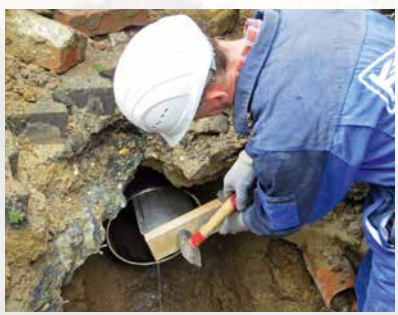
Connecting a PVC-U CONNEX pipe to a concrete pipe with a base using a BI-Adapter
