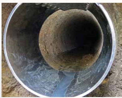
Connecting a PVC-U CONNEX pipe to a concrete pipe with a base using a BI-Adapter
