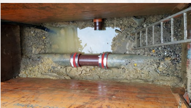
Subsequent integration of a repair branch (top) or repair pipe (below) in an existing vitrified clay pipe
