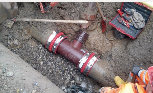
Subsequent integration of a repair branch (top) or repair pipe (below) in an existing vitrified clay pipe
