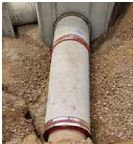
Sewer renovation with nominal diameter change
