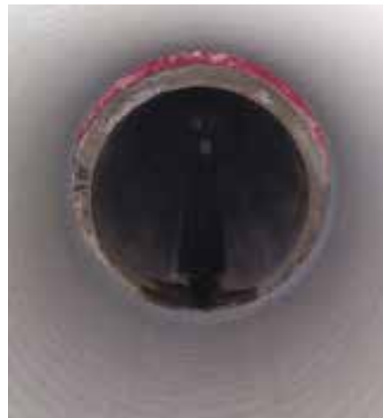
Professionally installed: The interior view illustrates the level invert.
