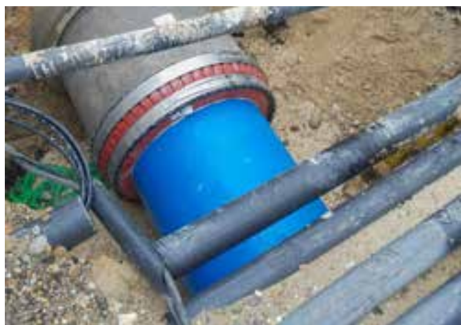
Connection of concrete pipe to HS® Pipe with different nominal widths
