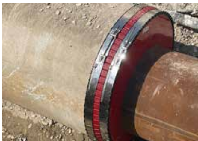
Reduction from a concrete pipe DN 1000 to a steel pipe DN 800
