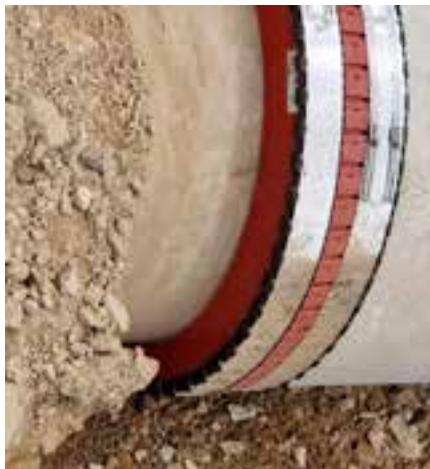
Upgrading an existing DN 700 concrete pipe to DN 800 concrete pipe.
